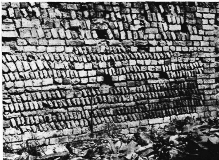
PLATE I. FIG. 1. EARLY BRICK WALLING Off Clarence Street, Dover.
